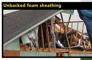
**The weak little triangle.** Foam sheathing performs better when the interior is covered with drywall. Gable ends without drywall, like the gables on these neighboring homes, should be sheathed with structural panels.
