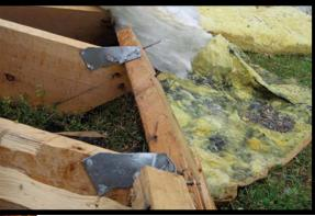
**Fastened, but not well enough.** This house's roof framing was attached to the walls' top plate with metal hurricane ties. Unfortunately, the ties were fastened on the inside of the top plate, where they aren't as strong as connectors aligned with the wall sheathing on the exterior.
