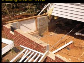
**Far from the foundation.** This house, which was attached to its masonry foundation with cut nails, was pushed 6 ft. off its foundation by tornado-driven wind. Similar failures occurred with houses that were nailed to slab foundations.
