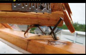
**Blown-away roof.** Unless it's adequately secured, roof framing can be pulled from the walls that it's attached to during high winds. Toenailed roof framing ripped from walls was the most commonly observed serious building failure in the author's poststorm research.
