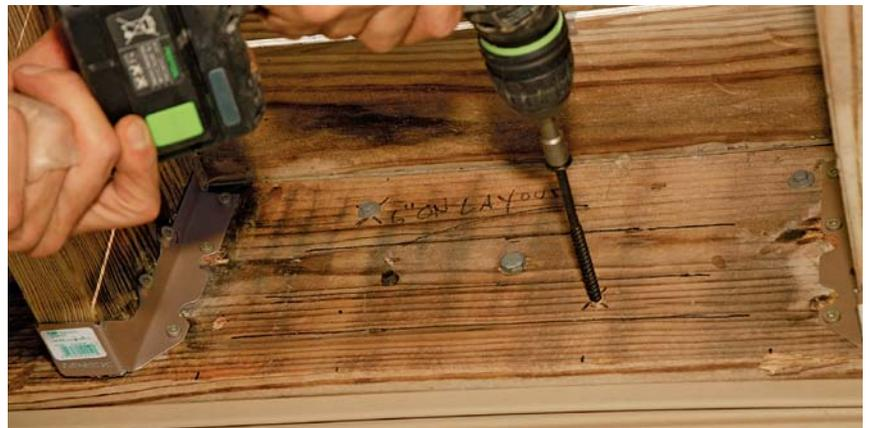
**Space new structural screws according to the manufacturer's installation table for the deck load and joist span.** These  $\frac{3}{8}$ -in. screws are long enough to penetrate through the ledger, the wall sheathing, and the house rim joist. They're staggered  $\frac{1}{4}$  in. from the top and bottom edges of the ledger and are doubled at the ledger ends and joints.
