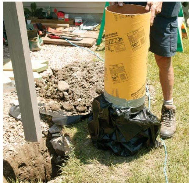
**A better footing.** After removing the old footings, dig the holes deeper and wider. Based on the footing-size table in DCA-6, footings need to be 16 in. dia. Local code specifies a 40-in. depth. On this job, the author used 12-in.-dia. form tubes with garbage bags taped to the bottom. The bags contain the concrete while permitting it to fill the 16-in.-dia. base entirely at the bottom of the hole. The bags also isolate the concrete from groundwater and soil contamination.
