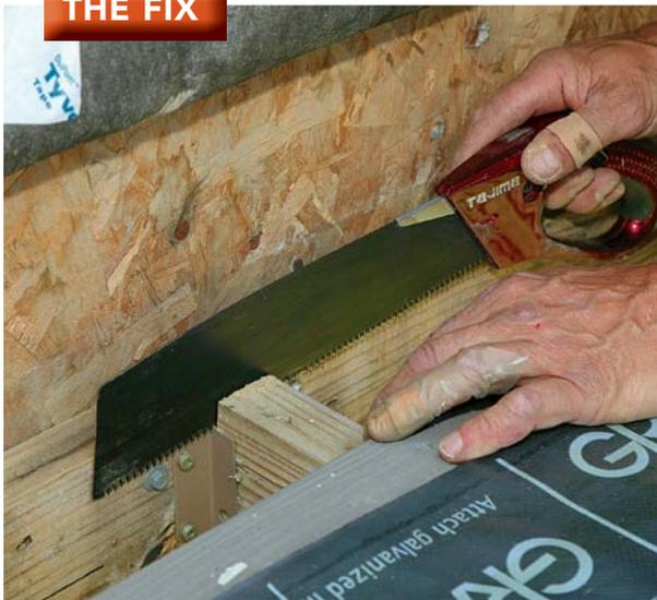
**Prepare for framing.** Remove the door riser board, the siding, and the first deck board to inspect for rot. After folding up the housewrap, cut a shallow kerf in the joist tops for the flashing edge.
