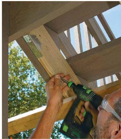
**Hardware reinforces the connection.** Screw galvanized stringer connectors (Simpson LSCZ or similar) to the header and to the new 2x6s to prevent the stringers from pulling away.
