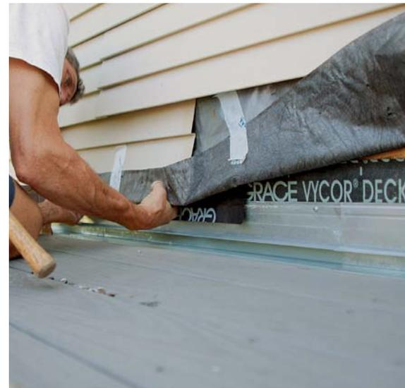
**Layers of protection.** After applying a strip of self-adhering membrane to the top of the ledger and onto the wall, install new flashing (everflashing.org) over the ledger. Counterflash the metal flashing with another piece of self-adhering membrane, and fold the housewrap back down over the wall leg.
