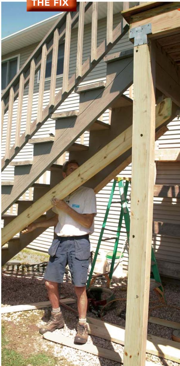
**Double up.** Issues of span, spacing, and overcut stringer notches can be resolved by sistering 2x6s along each stringer. To make it easier to fit them into place, cut the 2x6s short so that they can rest on ground-contact pressure-treated 4x4 blocks. Nail the 2x6s to the stringers with two rows of 12d galvanized nails, 12 in. on center.
