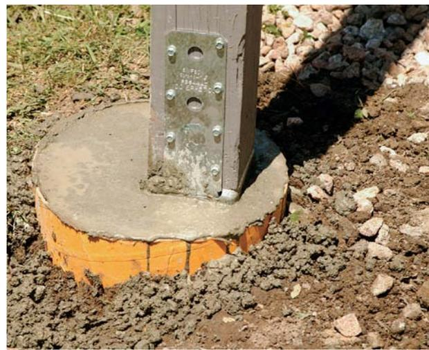
**Offset for a reason.** With the concrete in place, it's apparent that the post is not centered. The author offset the footing to make room for an additional post to support a new rim beam.
