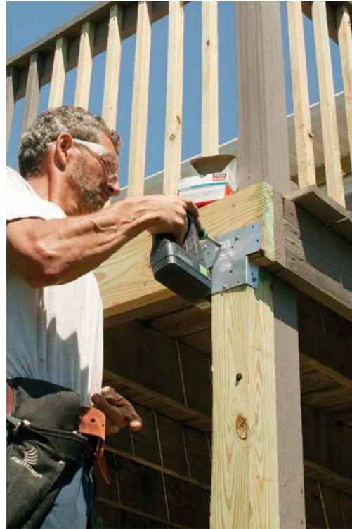
**Reinforce the span.** The single rim joist spans nearly 6 ft. between posts, far greater than allowed for the deck load. The DCA-6 beam-span table allows a maximum 6-ft. 2-in. span for a double 2x8 southern-yellow-pine beam that carries a joist span of 12 ft. After removing the outside decking board, nail a new rim to the existing rim with 16d galvanized nails; then secure each post-rim connection with a galvanized post cap (here, Simpson AC4Z).
