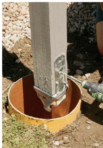
**Attach the hardware, then pour.** After locating and backfilling the tube, fasten the galvanized post base to the existing post.
