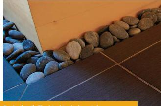
overflow drain. The hinoki tub doesn't have an overflow drain. To handle any water coming over the tub's rim, we set the tub, which has feet, in a sloped waterproof pan in the built-up floor. We filled the space between the tile and the tub with river stones. Any spills run through the stones to the drain below.
