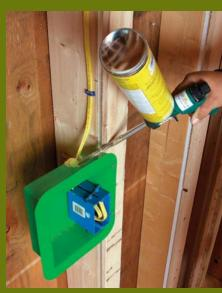
Install the enclosure and box. The green enclosure, which helps air-seal the electrical box, is nailed to the furring; then the electrical box is nailed to the plywood scrap. The last step is sealing the cables with foam.
