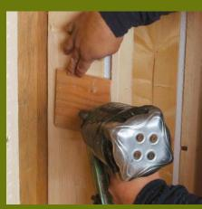
**Start with a plywood scrap.** A piece of <sup>3</sup>/<sub>4</sub>-in. plywood is nailed to the side of the stud to provide a solid installation point for the nail on electrical boxes.
