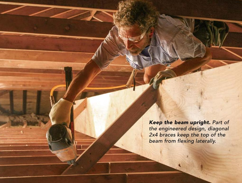
**Keep the beam upright.** Part of the engineered design, diagonal 2x4 braces keep the top of the beam from flexing laterally.
