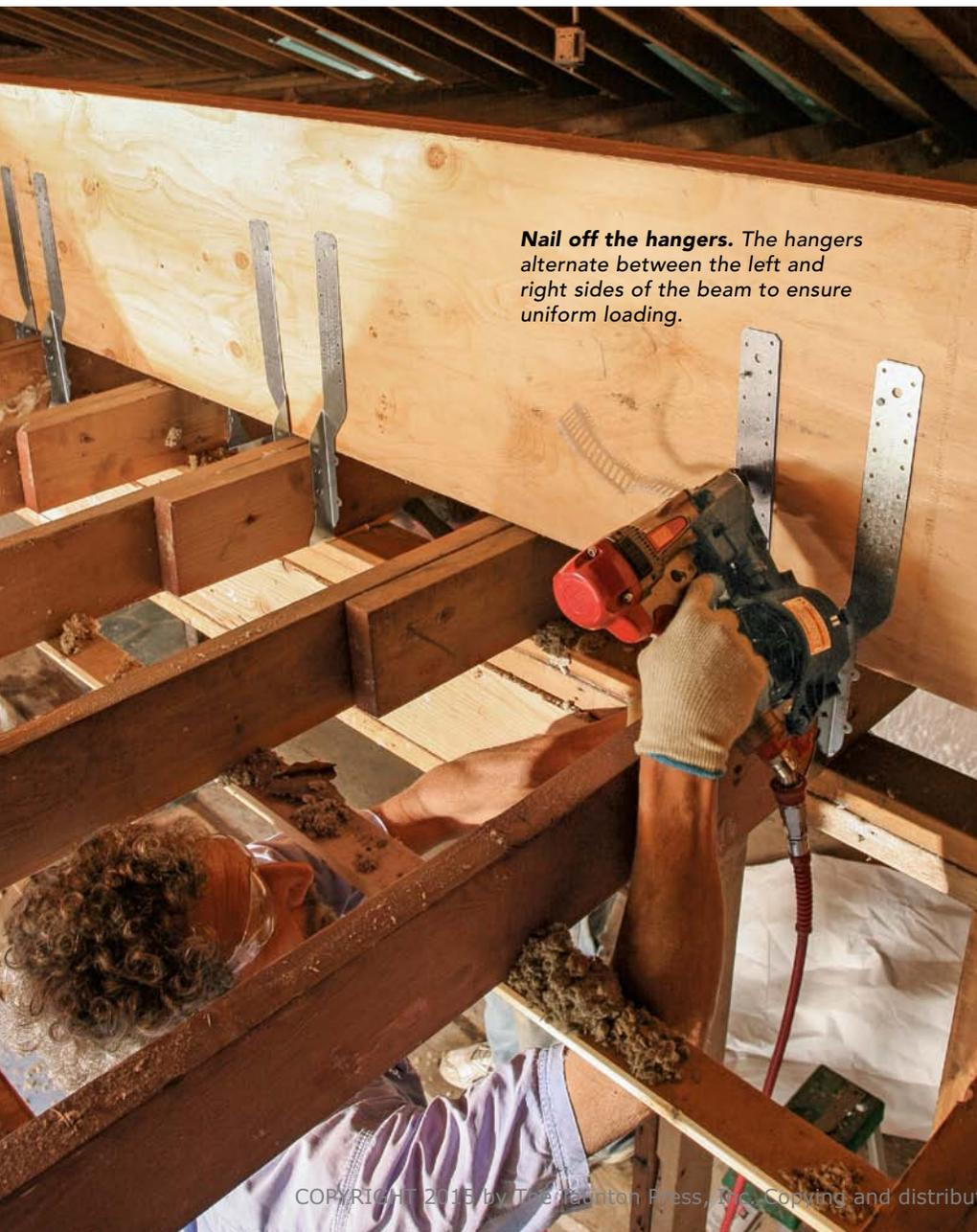
**Nail off the hangers.** The hangers alternate between the left and right sides of the beam to ensure uniform loading.
