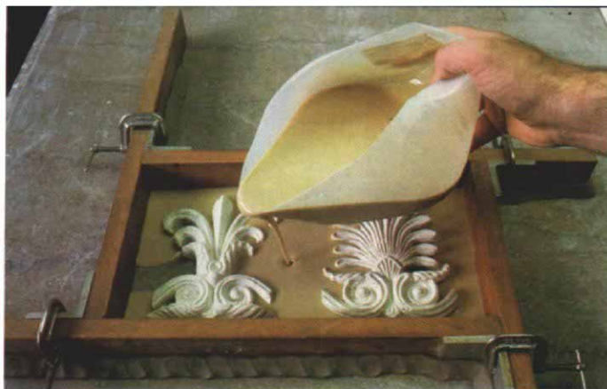
To make a flood mold, two-part urethane rubber is poured between wood fences clamped together and dammed with clay. The plaster models were first lathered with liquid soap (a parting agent). These pieces are for the parlor medallion.
