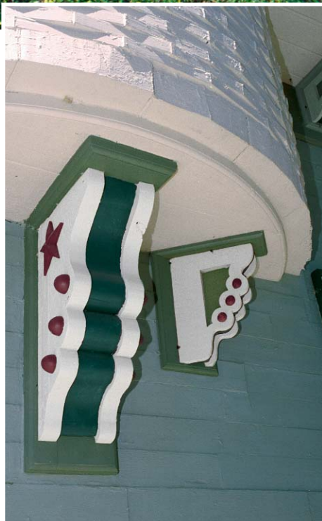
Fine home, low impact. Having recycled so much material, the author estimates that constructing this home required cutting only one new tree for lumber. The larger buttons on the corbels (photo left) are auto-body putty molded in eggshells. The smaller buttons, as well as the fretwork over the porch, are hickory shells.
