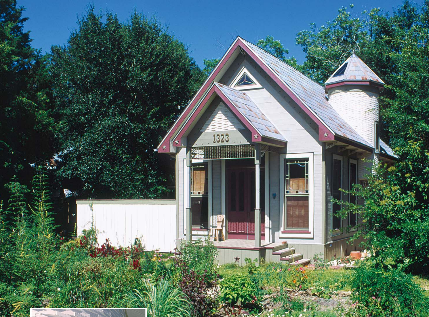
Fine home, low impact. Having recycled so much material, the author estimates that constructing this home required cutting only one new tree for lumber. The larger buttons on the corbels (photo left) are auto-body putty molded in eggshells. The smaller buttons, as well as the fretwork over the porch, are hickory shells.
