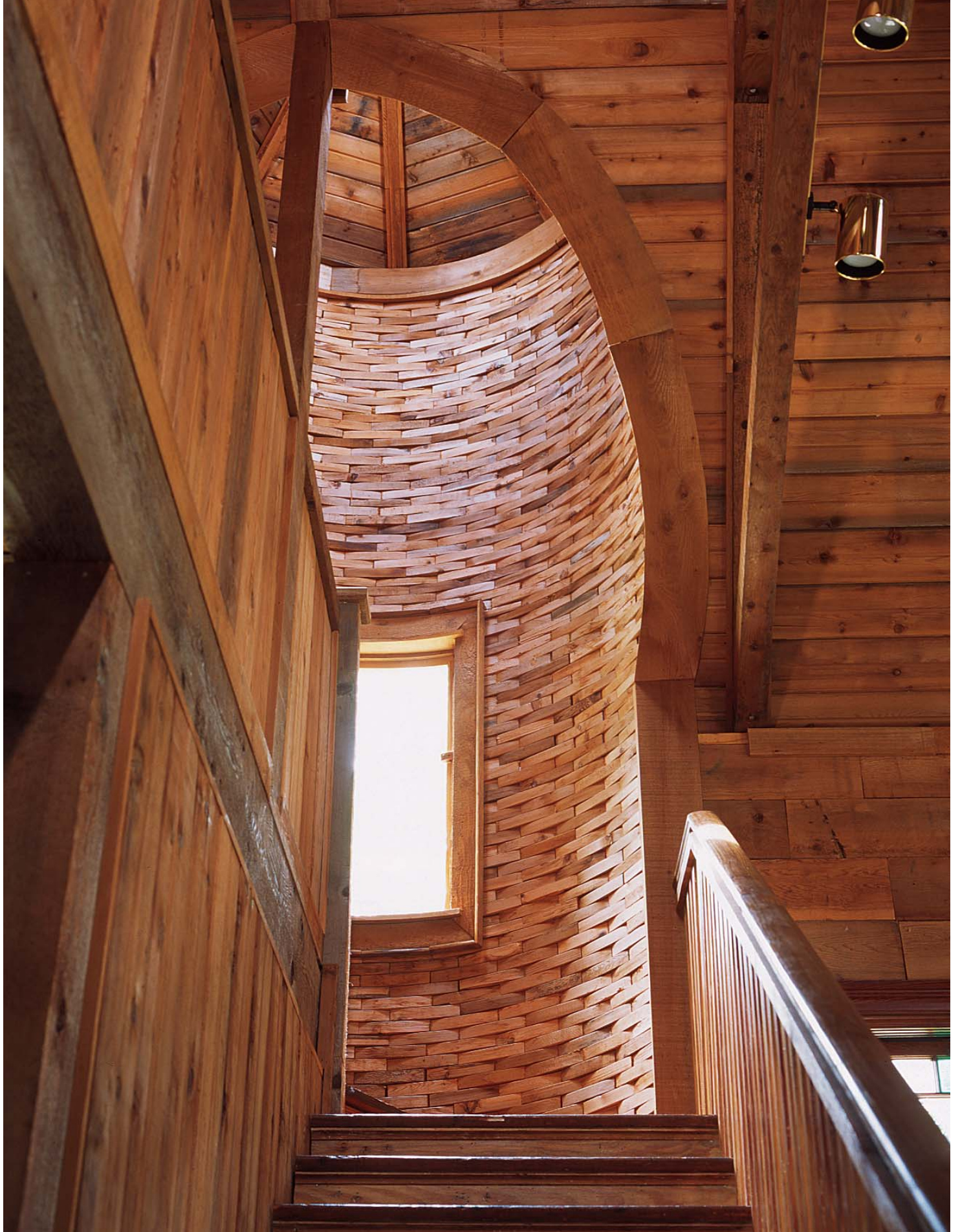
A basket-weave turret. The curved walls of this turret are made of 2x4 cutoffs, such as those shown on the facing page, stacked up like bricks. The stairs leading to the turret were salvaged intact from another house and delivered for $20.
