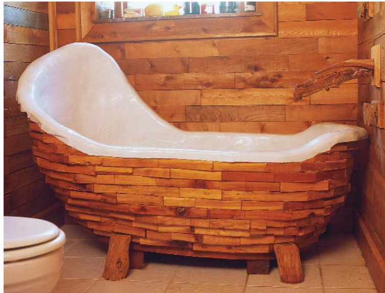
Not your average fiberglass tub. With a shell of 2x4 cutoffs, the author ground off interior edges and smoothed the surface with auto-body putty in preparation for two layers of fiberglass and epoxy paint.
