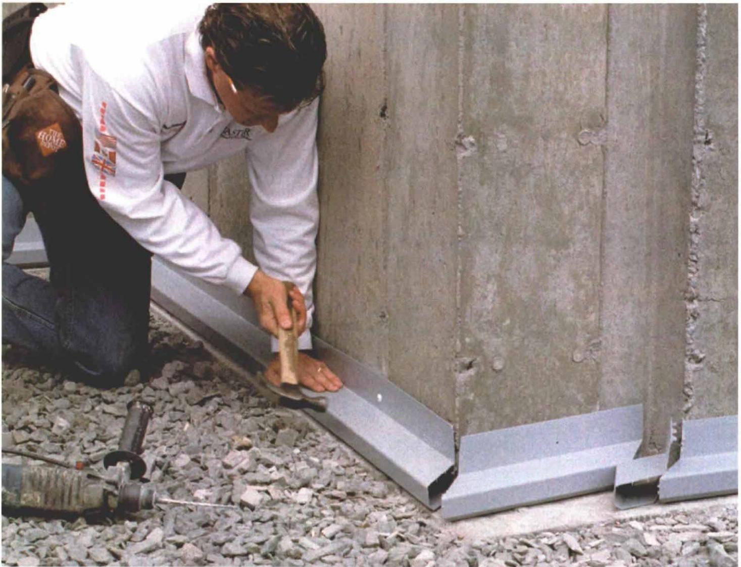
Interior perimeter drains are good insurance in new construction or retrofits. Plastic drains on top of the footing collect water that leaks in through the walls and channel it to the sump pump. The entire drain is to be covered with concrete, except the opening facing the wall.
