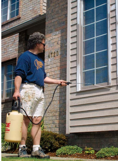
A garden sprayer makes a great chemical applicator. Prior to washing, a bleach-and-water solution is mixed in a garden sprayer and applied to the entire house to remove stains and to kill mildew. A garden sprayer is a lightweight alternative to the in-line chemical injector on the pressure washer.
