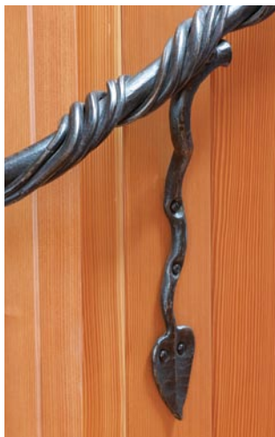
A handrail forged in fire. Sinewy, vinelike tendrils of hand-tooled steel wrap around the railing to the upper level. Glimpsed from the path, the Kimball house (top photo) is the epitome of a shelter in the woods: a gable roof and a chimney. Photo taken at A on floor plan.
