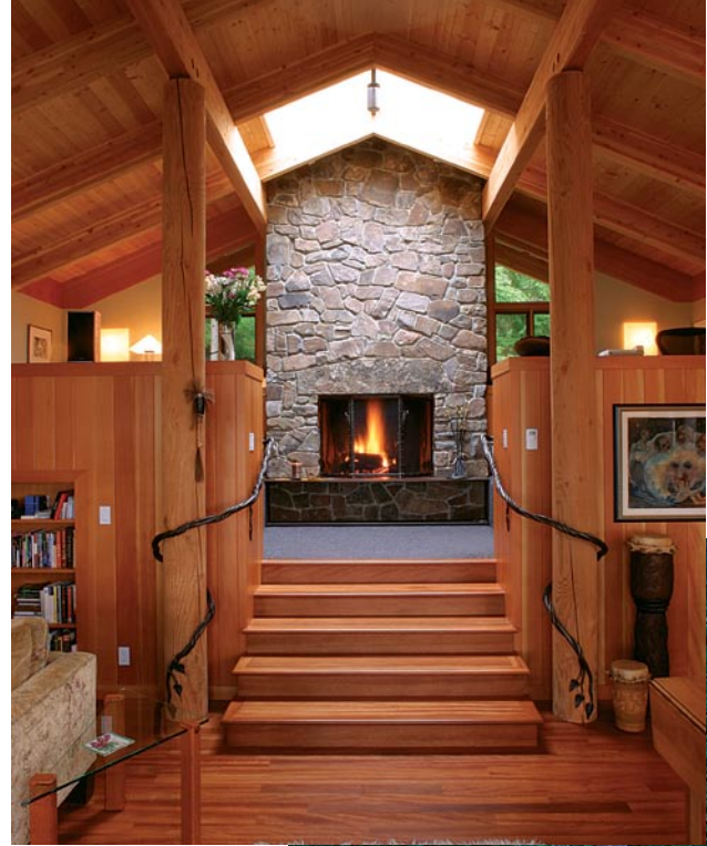
Complex on the inside. Centered on the ridge, a skylight pours raking light across the stone chimney and hearth. Note how the rafters cantilever over the beams adjacent to the chimney, eliminating the need for a light-blocking ridge beam. Photo above taken at B on floor plan.
