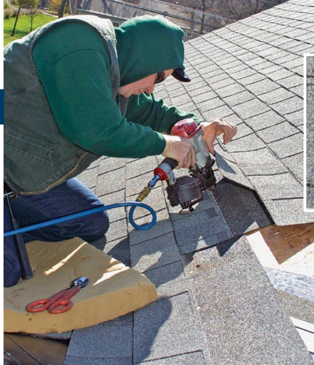
Typical nailing pattern: four nails per shingle
