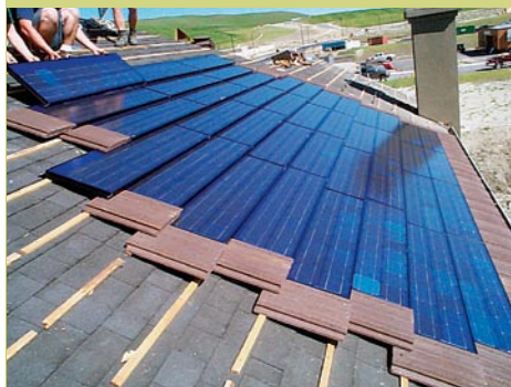
Photovoltaics are looking better all the time. Thin-film, high-efficiency solar panels that can be integrated into a house’s structure will increase consumer demand, which banks and local governments will fund with energy-related subsidies.
