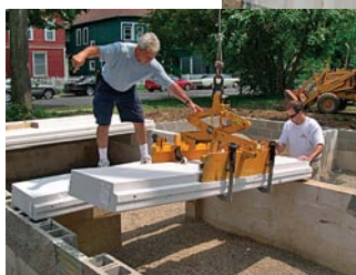
Modified concrete as the perfect material? The scarcity of wood and the need for more energy-efficient houses may drive builders to materials such as autoclaved cellular concrete. Extremely lightweight, the concrete mix can be cast into blocks or panels, is insectproof and energy-efficient, and can be cut with a circular saw. Photos courtesy of Aercon Industries.
