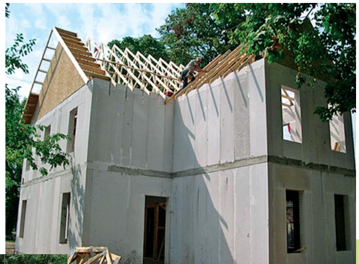
Modified concrete as the perfect material? The scarcity of wood and the need for more energy-efficient houses may drive builders to materials such as autoclaved cellular concrete. Extremely lightweight, the concrete mix can be cast into blocks or panels, is insectproof and energy-efficient, and can be cut with a circular saw. Photos courtesy of Aercon Industries.
