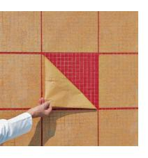
ic consistency and applied to an exacting depth so that the tiles bond properly. Also, cracks are more visible on glass tiles, necessitating special cutting techniques and sometimes requiring a crack-suppression membrane, which prevents shrinkage and movement of the substrate.
