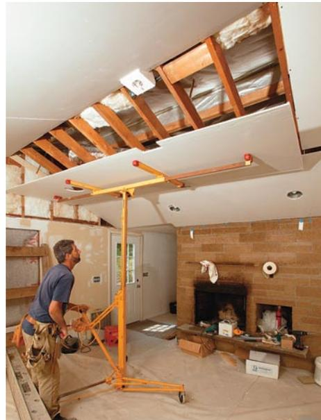
**Rent a helper.** Drywall lifts are usually available at local rental outlets and are worth every penny. They save time and make solo installation of even a 12-ft.-long sheet an easy task. With the addition of skylights (photo below), the finished ceiling adds light and space to the living room.
