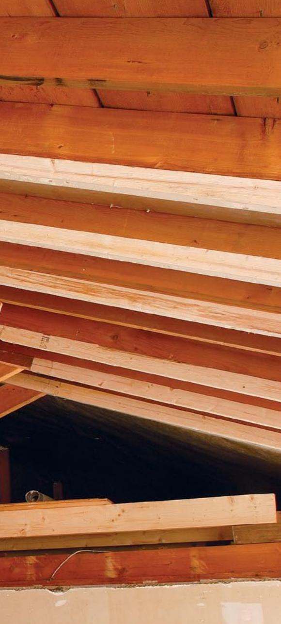
joists to the plates; this process prevented the joist ends from splitting. Once the nails had been removed, the strapping and the joists would provide much of the lumber needed to frame the new ceiling.
