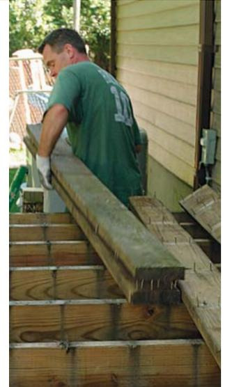
**Quick and safe board removal.** When headed to the Dumpster, instead of bending over nails or pulling them out, carry two boards together with the protruding nails facing each other.
