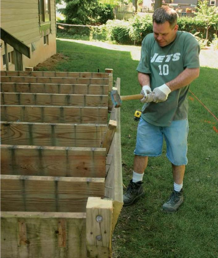
**Just beat it.** Sometimes the solution really is to use a bigger hammer. A sledge can make quick work of removing a rim joist, which is often held in place only by nails driven into the end grain of the joists.
