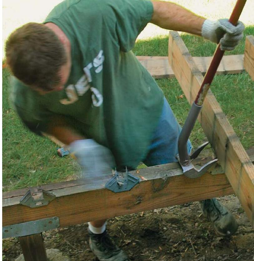
**Remove joists in a two-step process.** On a low deck like this, pry each joist off the beam (above), and then lever the other end out of the joist hanger attached to the ledger (inset).
