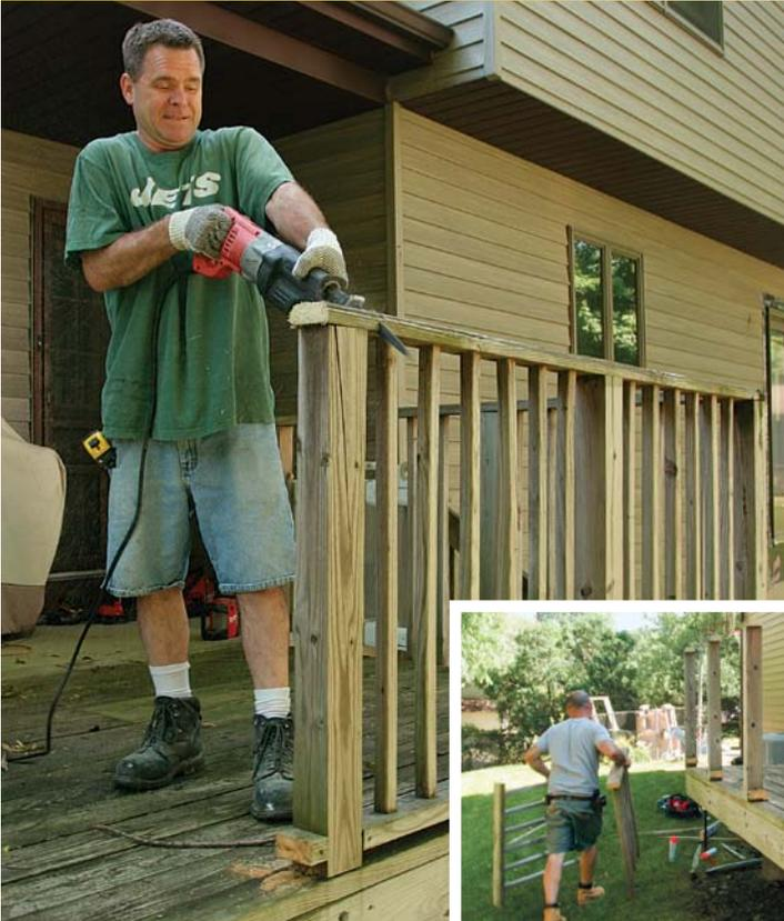
**Cut the railing.** Cut a few inches from where the railing meets the post so that you don't hit any nails, leaving a stub of railing on the post. Clear the debris as you work so that you don't trip.
