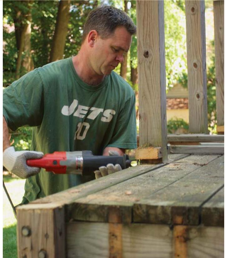
**Don't unbolt—just cut.** A pruning blade in a reciprocating saw makes fast work of cutting the railing posts free from the deck.
