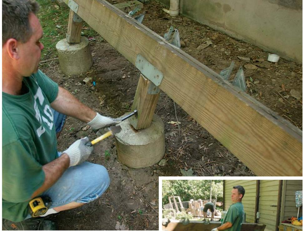
**Pull nails only when necessary.** A taller deck's longer posts would have levered out of the post bases. In this case, the hardware's nails had to be pulled using a cat's paw.
