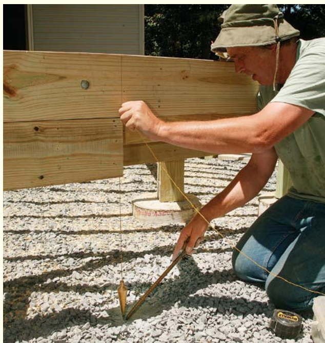
Locating the bottom frame. The skirt frame consists of a kerfed 2x4, top and bottom. After the top 2x4 is attached to blocking, a plumb bob establishes the position of the bottom half of the frame.
