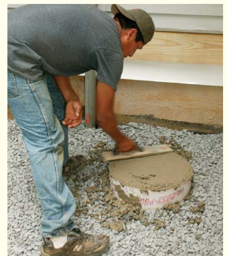
Prep for the next step. Once the footing is poured, a wooden float is used to screed off the excess so that the concrete is flush with the top of the footing form.
