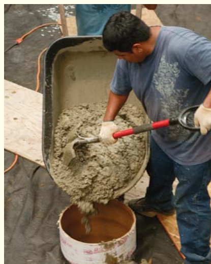
The truck won't reach. Due to limited access to the site, the crew has to transfer the concrete from the truck to a wheelbarrow. Plywood pathways make it easier to roll between the truck and the footings.
