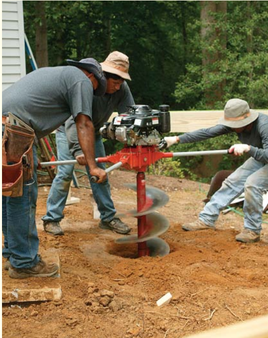
Hang on. Nominally a two-man machine, the aggressive auger sometimes required three operators as it dug into the hard-packed soil. The auger rental saved time and money.
