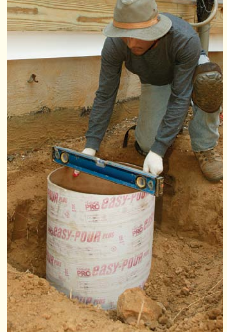
Plumb the footings. A short level held across the top indicates when the form is level and, therefore, plumb. When the forms are plumb, they are backfilled.
