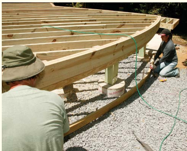
Pins determine the curve. The 12-in.-long rebar pins are driven into the ground below the upper frame, and the lower frame is bent around them. The lower frame is secured with more pins driven through pilot holes drilled every 2 ft. along the width of the 2x4.
