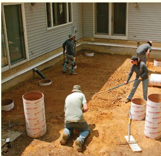
Dig, fill, and clean up. As the builder's forms are placed and backfilled, the site is raked to slope away from the house in preparation for a layer of landscape fabric and gravel beneath the deck. The gravel minimizes moisture transpiration and creates a safer working surface.
