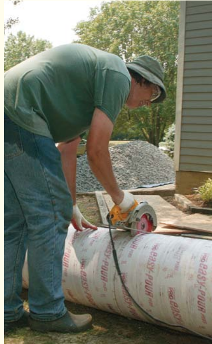
Form prep, production style. The easiest way to cut cardboard footing forms to length is to use a circular saw while a helper rotates the form. The cuts should be as square as possible.
