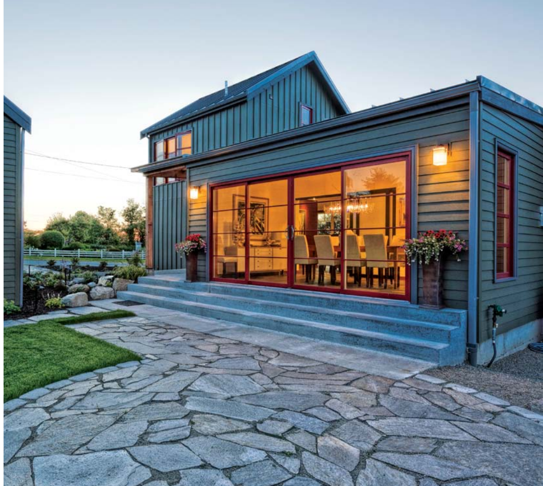
Sunlight and shelter. A central patio is sheltered from the wind by the structures around it. Sunlight passing through the south-facing dining-area doors is stored by the thermal mass of the tile-and-concrete floor.
