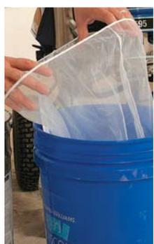
**Stir and strain.** Fully mix the paint in accordance with the product instructions, and strain it through a mesh strainer bag into a clean container. Add more paint than you think you'll need. You can pour any excess back during clean up.
