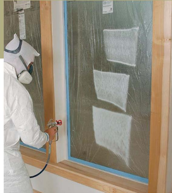
**Adjust the pressure.** Use the lowest pressure that fully atomizes the paint. Make a test spray on the masking materials, and gradually increase the pressure until there are no small lines, called "fingers," at the top and bottom of the spray pattern. If you see fingers, increase the pressure until the spray pattern shows full and even coverage across its width.
