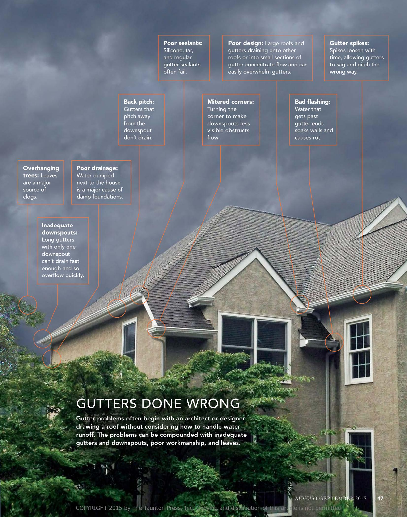
**Poor sealants:** Silicone, tar, and regular gutter sealants often fail.
