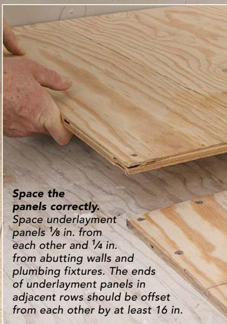
**Space the panels correctly.** Space underlayment panels  $\frac{1}{8}$  in. from each other and  $\frac{1}{4}$  in. from abutting walls and plumbing fixtures. The ends of underlayment panels in adjacent rows should be offset from each other by at least 16 in.
