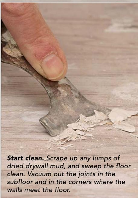
**Start clean.** Scrape up any lumps of dried drywall mud, and sweep the floor clean. Vacuum out the joints in the subfloor and in the corners where the walls meet the floor.
