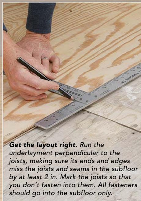
**Get the layout right.** Run the underlayment perpendicular to the joists, making sure its ends and edges miss the joists and seams in the subfloor by at least 2 in. Mark the joists so that you don't fasten into them. All fasteners should go into the subfloor only.
