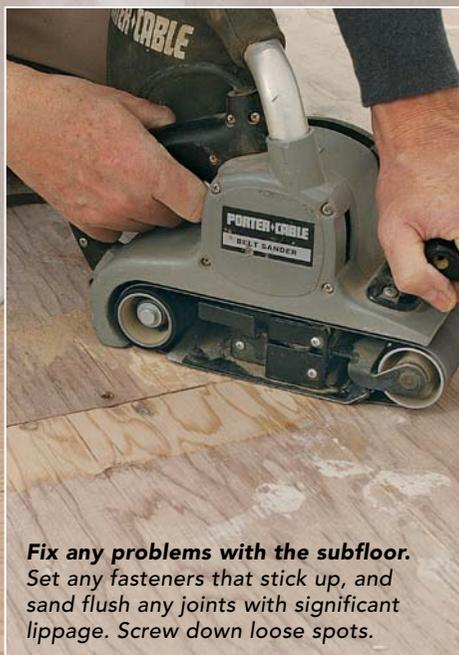
**Fix any problems with the subfloor.** Set any fasteners that stick up, and sand flush any joints with significant lippage. Screw down loose spots.
