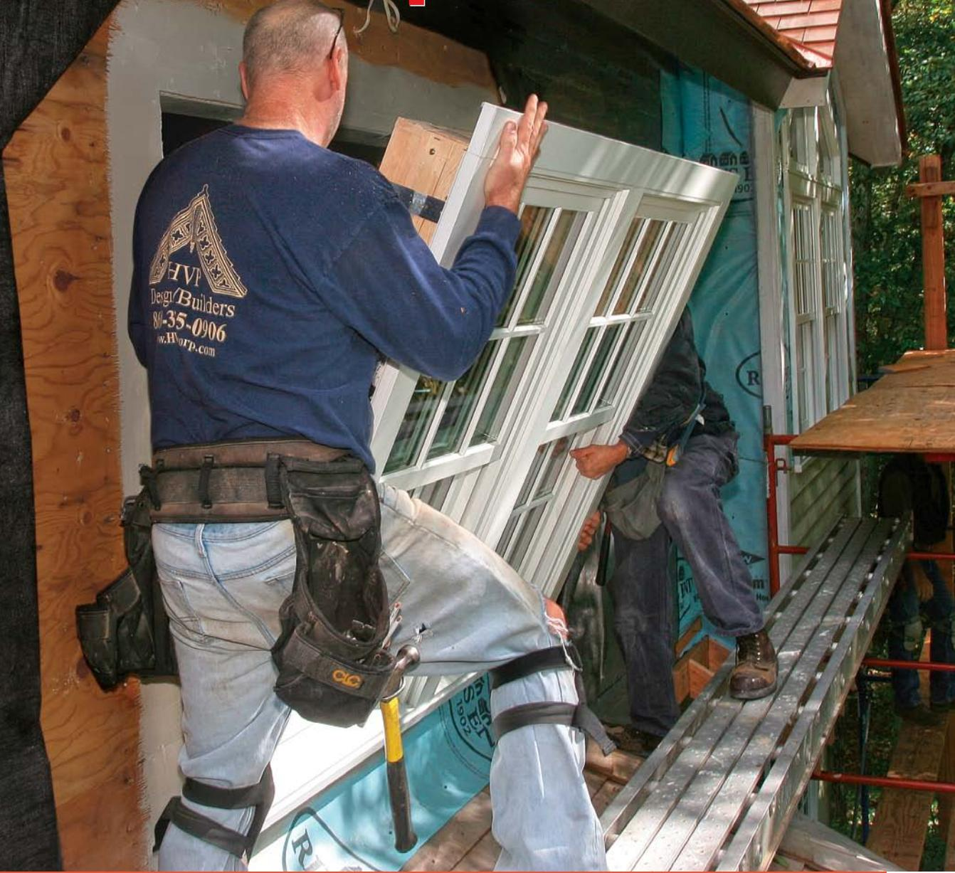
**Brush-on membrane speeds window flashing.** In most cases, a mechanical connection such as flashing tape is used to bridge the rough opening and the housewrap. LAF application methods vary, with some products brushed on (shown) and others applied with
