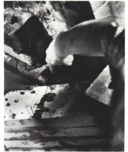
When the fireback is only one brick long, the most efficient way to butt-cove and fireback is to cut the coving brick to fit along the fireback's header, left. When the fireback is longer, cut the coving brick to fit against fireback stretchers. Above, firebox is filled in behind with rubble and masonry. A fairly wet concrete mix will flow to the bottom.
