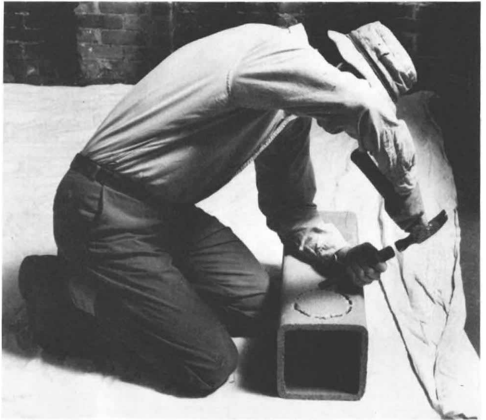
The first section of liner is cut to receive the thimble fitting, a tricky business since the ceramic material is very brittle. Closely spaced holes are first drilled along the cut-line; then the waste piece is knocked out with a hammer and chisel, as shown.
