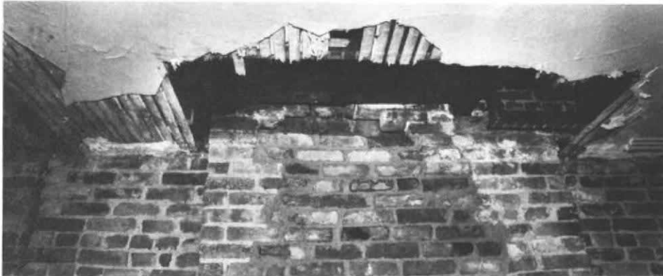
A round flue section is cemented to the square base, left. To ensure a good fit, a square piece of wire lath with a hole cut in the middle is set in the mortar between the two liners. Right, joints between round liner sections are sealed completely with mortar. The remaining interior brickwork extends to within an inch or so of the liner, allowing room for heat-induced expansion. Face ties in the last interior course will be bent into the face course as the wall is rebuilt.
