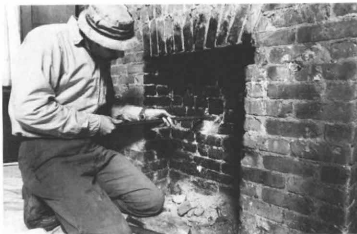
The first step in installing new flue liners is removing bricks from the second-floor fireplace to expose the chimney cavity. Hammer, railroad spike and pry bar are essential tools. A vinyl-covered canvas dropcloth over rubber carpet padding protects the floor. At right, Kitchel aligns two pieces of angle iron, which will be cemented in place across the face of the cavity to reinforce the chimney before the new liner is installed.
