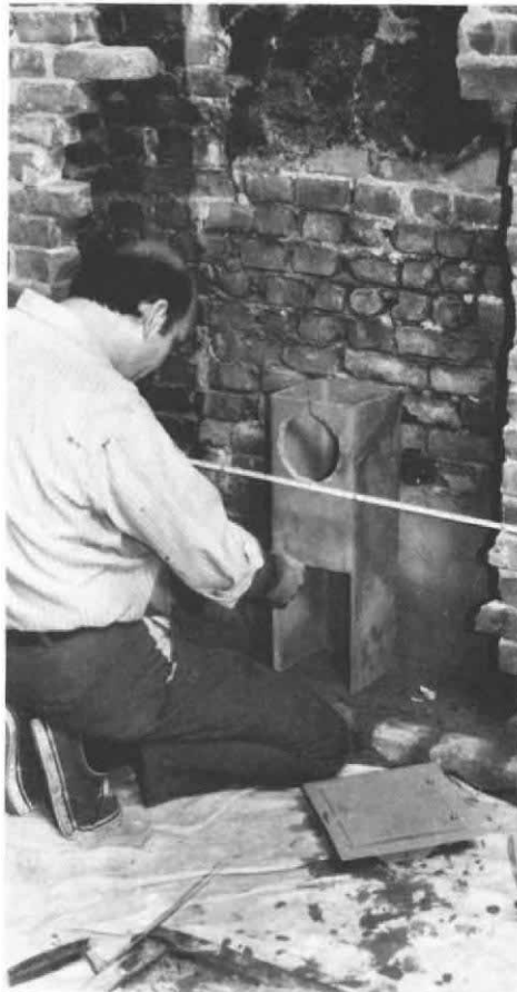
After the cavity has been built up to floor level, the first flue section can go in, left. The square opening at the bottom of the flue will receive the cleanout fitting. When both flue sections are in place, the chimney is bricked in around them, starting with a layer of cement blocks, right. The round flue section will eventually be connected to a new lining from the floor below; the square section in the foreground is for the second-floor lining. The back walls of old chimneys like this one usually require parging, or stuccoing over, before the new lining and interior brickwork can be laid in.
