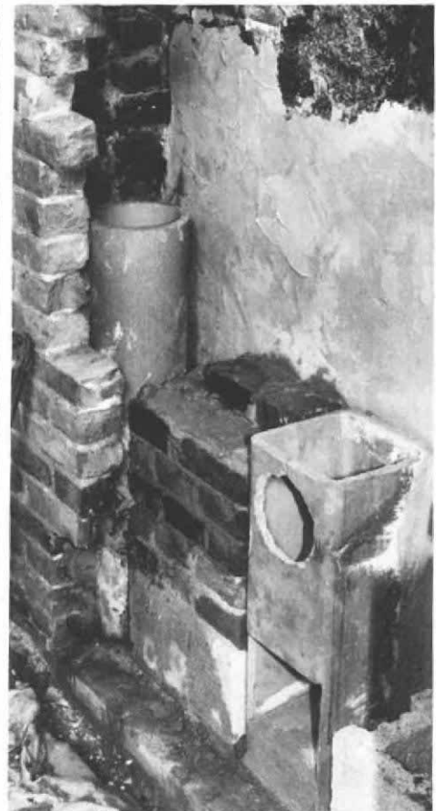
After the cavity has been built up to floor level, the first flue section can go in, left. The square opening at the bottom of the flue will receive the cleanout fitting. When both flue sections are in place, the chimney is bricked in around them, starting with a layer of cement blocks, right. The round flue section will eventually be connected to a new lining from the floor below; the square section in the foreground is for the second-floor lining. The back walls of old chimneys like this one usually require parging, or stuccoing over, before the new lining and interior brickwork can be laid in.
