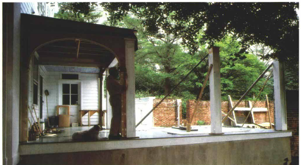
Nailing strips are fastened to the ceiling and new column sides (left) in preparation for attaching one plywood face of the entablature. Right, two identical plywood arches, fastened to nailing strips and joined with a curved soffit, complete the entablature between columns. Repeating this motif will connect the two additional columns on the finished porch, making a colonnade.
