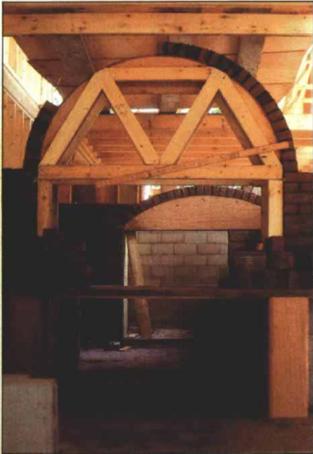
D. The ends of the bricks in the arch must be in the same plane as the wall. Check for alignment with a trammel board tacked to the center of the horizontal truss member.
