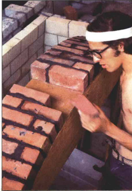
E. Bricks are set between the pencil lines that were drawn on the centering during a test-fitting on the ground. This guarantees a proper fit and mortar joints of uniform size.
