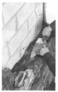
Balance and alignment. At right, stone chips inserted along joint lines to serve as temporary wedges prevent tall, thin stones from leaning out of plumb. They're removed after the mortar has set. The facing is thick enough to conceal a heating duct in the wall. Below, corner and curve construction depends on a good selection of shapes and sizes. A mixture of small and large stones also makes it easier to stagger the joint lines.
