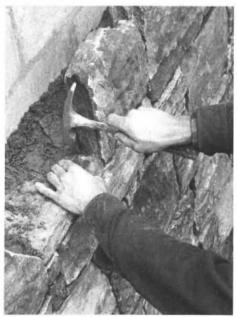
Hiding the mortar. The key to the dry-fit appearance is to keep mortar away from the face edge of each joint. Neufeld packs the mortar close to the block, left, then presses the stone in place and seats it in its mortar bed with several hammer blows, as shown above.
