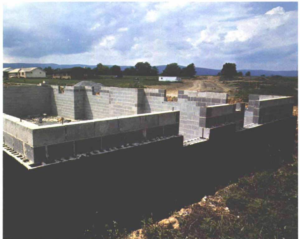
The completed foundation has been sealed with two 1/4-in. thick parging coats and topped with an application of tar compound, which finishes the waterproofing. Backfilling should happen only after the first floor is framed and the walls framed up, so the added weight of the structure will stiffen the walls and make them less liable to bulge from the pressure of the earth.
