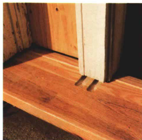
The new sill was splined together from two pieces of 10/4 oak, cut to the dimensions and angles shown in the drawing. The double mortises in the sill received the tenons at the bottom of the door jambs (photo left). Once the sill was in place, the pilaster bases were reinstalled (photo right), using shims to close up the joints between the middle and top half-round sections. The slivers that were cut out of the pilaster so that the sill could slide in were later glued back in place.
