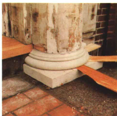
The new sill was splined together from two pieces of 10/4 oak, cut to the dimensions and angles shown in the drawing. The double mortises in the sill received the tenons at the bottom of the door jambs (photo left). Once the sill was in place, the pilaster bases were reinstalled (photo right), using shims to close up the joints between the middle and top half-round sections. The slivers that were cut out of the pilaster so that the sill could slide in were later glued back in place.
