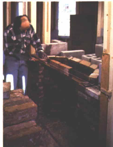
The lintel. Side walls, back wall, and angle-iron lintel are at the same height to support the damper. The first course of bricks over the lintel overhangs the flange of the angle iron, and these bricks have to be laid up carefully so they won't roll forward. Pieces of building paper tucked at the ends of the angle iron serve as expansion joints.
