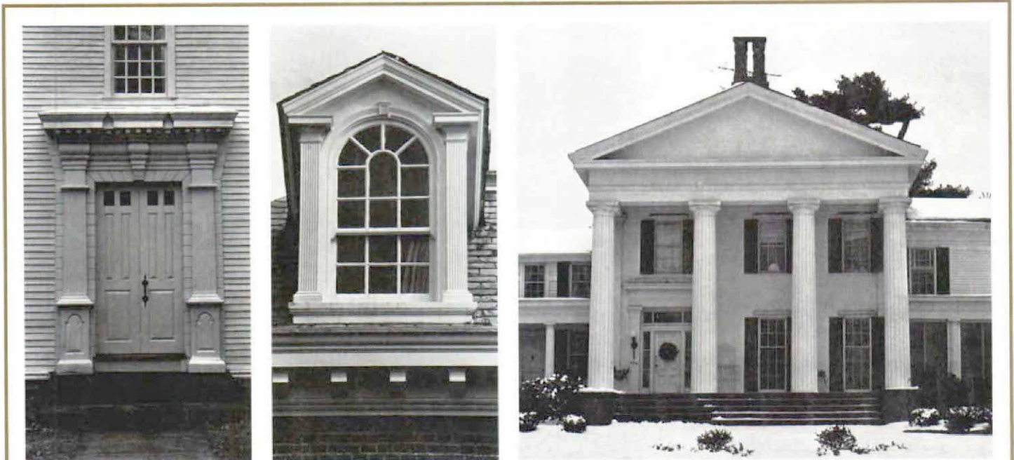
Georgian entrances were often elaborate, formal and robust. Builders imitated Roman moldings, and based their details on segments of the circle.
