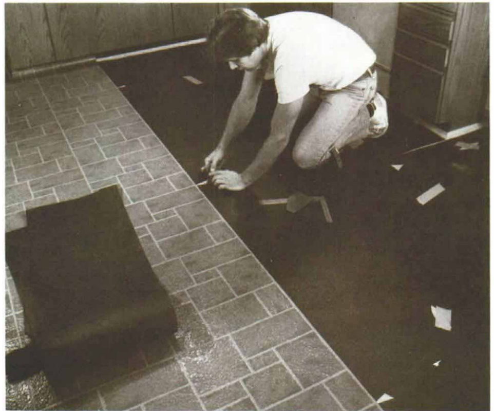
Shrode uses notches cut in the pattern felt to register the second drop to the first. The notches are placed three design repetitions apart, and let him accurately position the pattern on the material.
