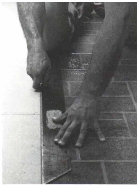
Sheet goods are made extra wide and have to be trimmed at the seams. The author prefers to cut one sheet at a time, using a long straightedge and a utility knife to score the vinyl, left. The cut is finished with a linoleum knife, above.
