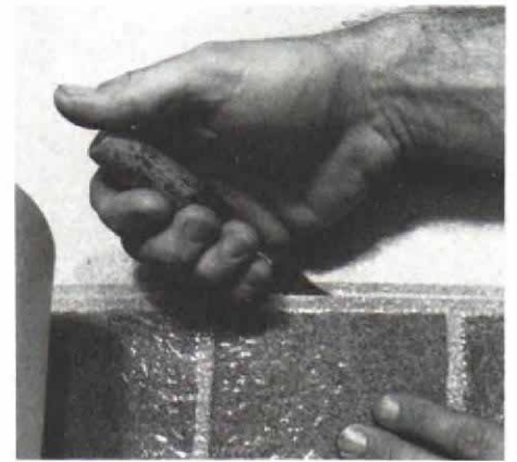
Sheet goods are made extra wide and have to be trimmed at the seams. The author prefers to cut one sheet at a time, using a long straightedge and a utility knife to score the vinyl, left. The cut is finished with a linoleum knife, above.
