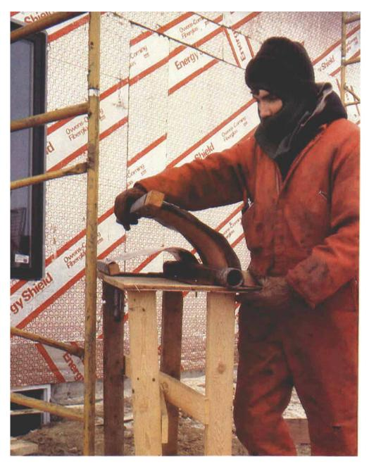
leys, hips and gables. We call these gable-bent shingles. This is the easiest type of bend to make, and some shingles are flexible enough to be bent and nailed without steaming.
