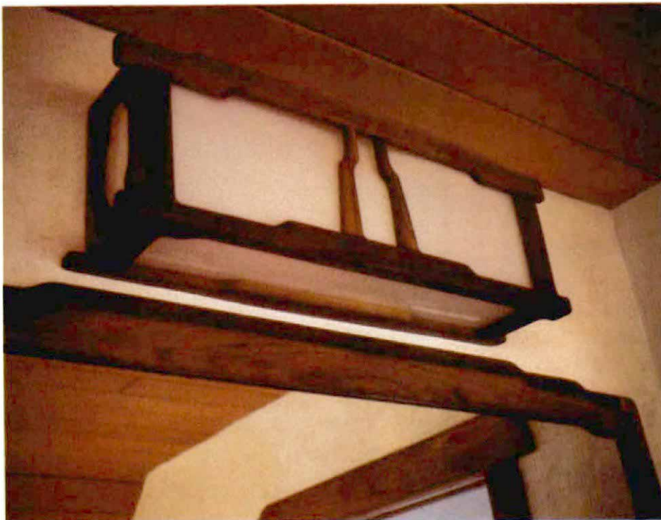
Lasso built the wall bracket above using the techniques detailed in the drawing at top. Housing the plastic panels in slots solves potential shrinkage problems.
