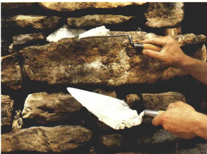
Pointing. A rich, buttery mix of pointing mortar made with fine sand sits well on the trowel and is easy to work. At left, Kennedy uses a pointing trowel to work the mortar into joints between stones. When the mortar starts to dry, he goes over it with a stiff, dry brush, right, smoothing the joint tight against the stones and brushing away small splatters and crumbs. Pointing mortar should be kept damp to prolong its curing time.
