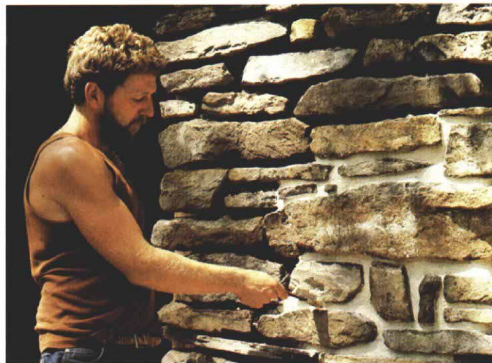
Pointing. A rich, buttery mix of pointing mortar made with fine sand sits well on the trowel and is easy to work. At left, Kennedy uses a pointing trowel to work the mortar into joints between stones. When the mortar starts to dry, he goes over it with a stiff, dry brush, right, smoothing the joint tight against the stones and brushing away small splatters and crumbs. Pointing mortar should be kept damp to prolong its curing time.
