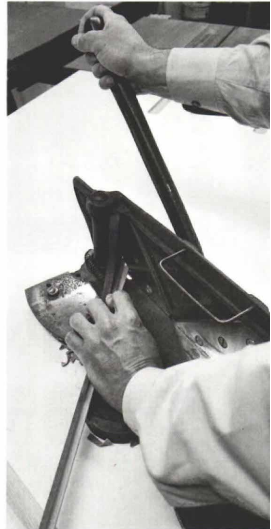
To miter the solid wood lipping that covers the edges of the doors and drawers, Levine uses a razor-sharp picture framer's trimmer, above. An accurate choppersaw with a finish-cutting blade will also work. Details of flush-fit cabinet construction are shown in the drawing, facing page.
