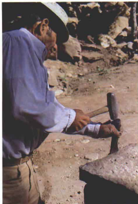
A pitching chisel is used to remove unwanted material in a hurry. Here Soto uses one to clean up a ragged edge on a flagstone.
