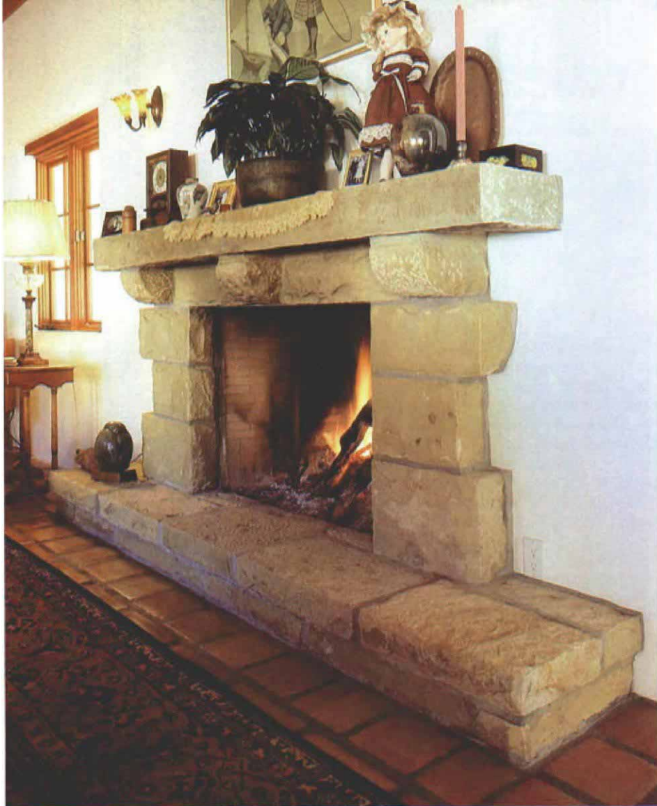
The weighty presence of hand-wrought stonework is entirely in keeping with the sturdy detail in this Spanish Colonial Revival style home. Soto used a plywood template to regulate the curvature on the bottoms of the corbels that support the mantel, and he shaped them with a pitching chisel.
