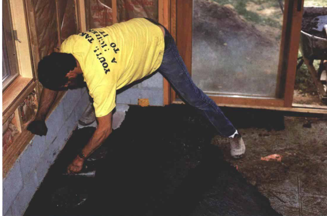
After the flue-run lids were complete, Marcus laid in rebar and installed two 8-in. cleanout ducts with airtight lids (left). He also laid in a 3-in. aluminum pipe wrapped in fiberglass that was intended to heat cold air from the basement. Marcus added black dye to the concrete for the finished slab (above) in order to increase the absorption of winter-time solar heat. The k'ang, finished except for an airtight firebox door, is shown below. Photos above: Jeffrey Smith.
