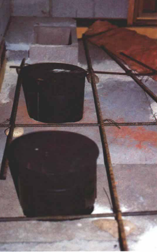
After the flue-run lids were complete, Marcus laid in rebar and installed two 8-in. cleanout ducts with airtight lids (left). He also laid in a 3-in. aluminum pipe wrapped in fiberglass that was intended to heat cold air from the basement. Marcus added black dye to the concrete for the finished slab (above) in order to increase the absorption of winter-time solar heat. The k'ang, finished except for an airtight firebox door, is shown below. Photos above: Jeffrey Smith.
