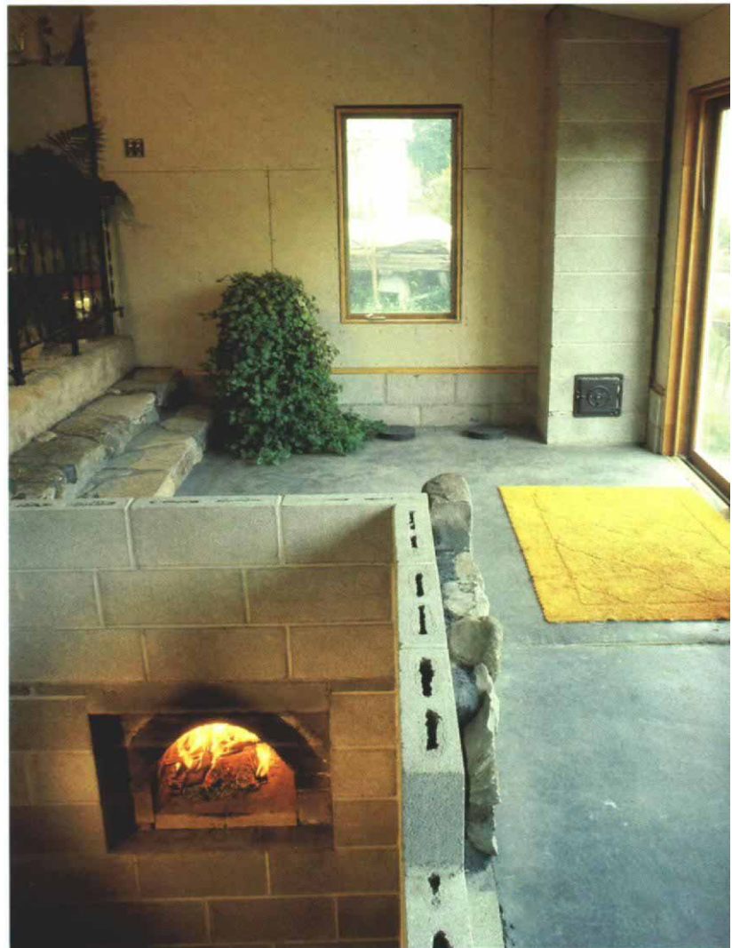
After the flue-run lids were complete, Marcus laid in rebar and installed two 8-in. cleanout ducts with airtight lids (left). He also laid in a 3-in. aluminum pipe wrapped in fiberglass that was intended to heat cold air from the basement. Marcus added black dye to the concrete for the finished slab (above) in order to increase the absorption of winter-time solar heat. The k'ang, finished except for an airtight firebox door, is shown below. Photos above: Jeffrey Smith.
