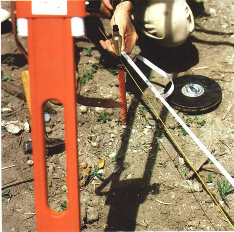
Once the temporary stake is in the ground to establish alignment, a measurement can be made by pulling a steel tape between the new stake and a known corner such as this one.
