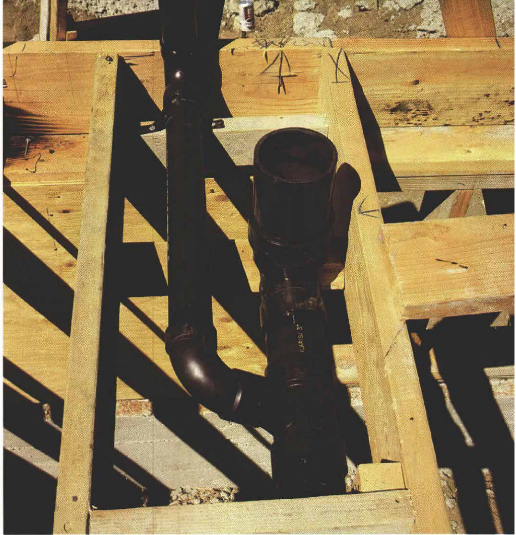
Alignment is critical. The mark on the joist to the right of the water-closet drain stub in the photo above shows the closet flange centerline from the wall. Above it, the X marks the line of the wall. The tub p-trap (photo below) was positioned after the bathtub was in place. Most bathtubs have a skirt that conceals the floor behind them, so you can cut a fairly large hole in the floor to make it easier to align the fittings.
