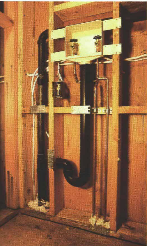
A recessed laundry box organizes the washing-machine supply lines and drain. The drain stack in the lower left corner is the extension from the downstairs bathroom in the photo at the top of the page. Urethane foam fills the gaps around the pipes at the plates, securing the pipes and cutting air infiltration.
