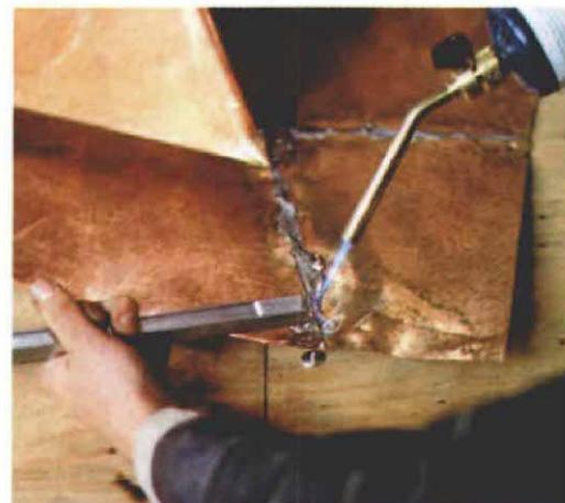
**McBride solders the flashing in his shop, instead of on the roof. This way he can position the flashing so that the seams are level when he solders them, which keeps the molten solder from running out of the joint.**
