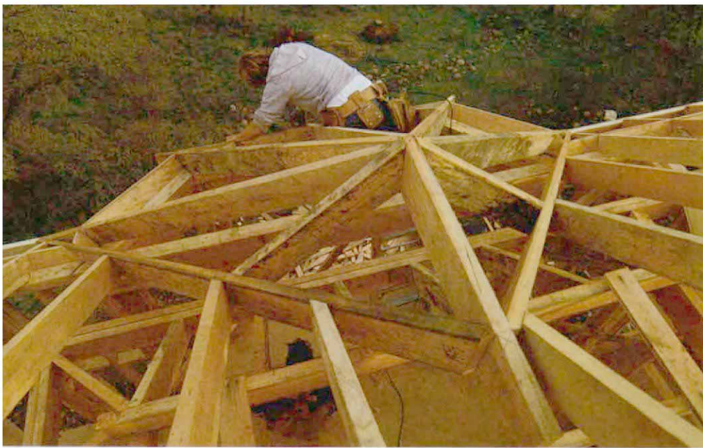
Converging rafters meet at the end of the bay's ridge beam. In the lower left corner of the photo you can see where the valleys intersect the ridge. The "X" marks one end of the 2-ft. ridge.
