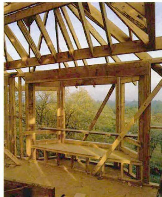
The author nails down irregular hip rafter A on a cantilevered bay (photo below). Note the 1x4 king studs in the diagonal walls. They allow more room for the window. Opposing walls are joined by a tie beam across the top of the opening to the bay (photo above). The upper half of the top plate has been let into the beam for several feet.
