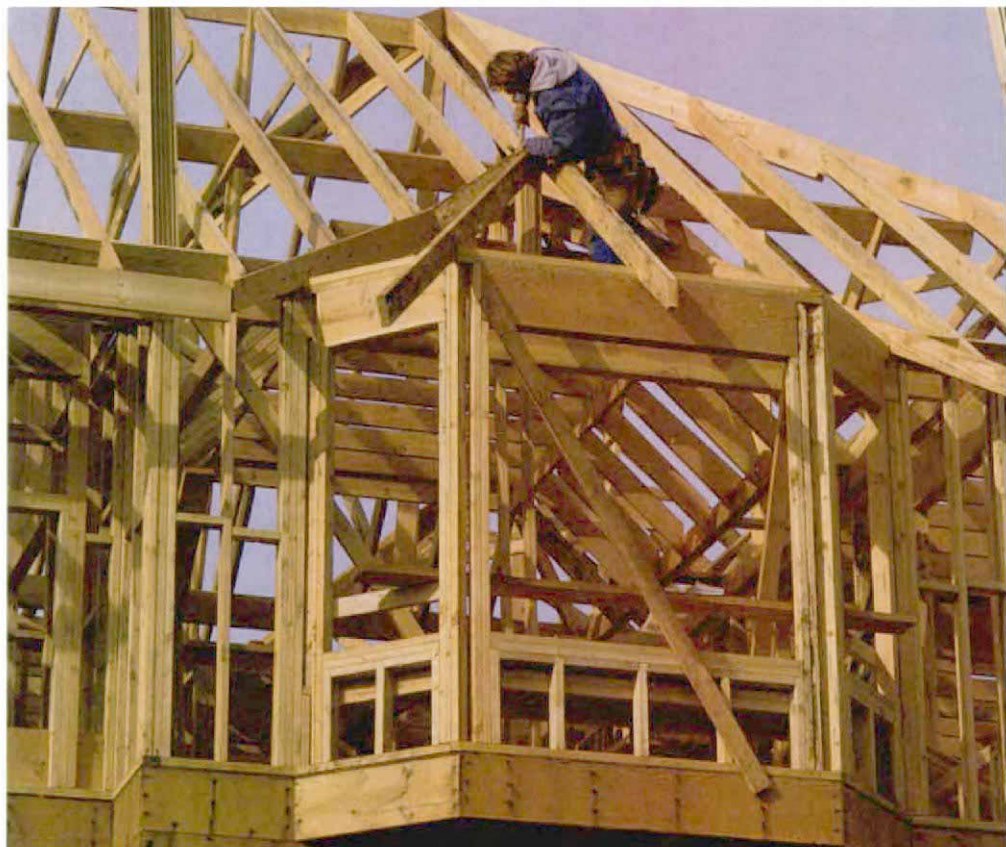
The author nails down irregular hip rafter A on a cantilevered bay (photo below). Note the 1x4 king studs in the diagonal walls. They allow more room for the window. Opposing walls are joined by a tie beam across the top of the opening to the bay (photo above). The upper half of the top plate has been let into the beam for several feet.
