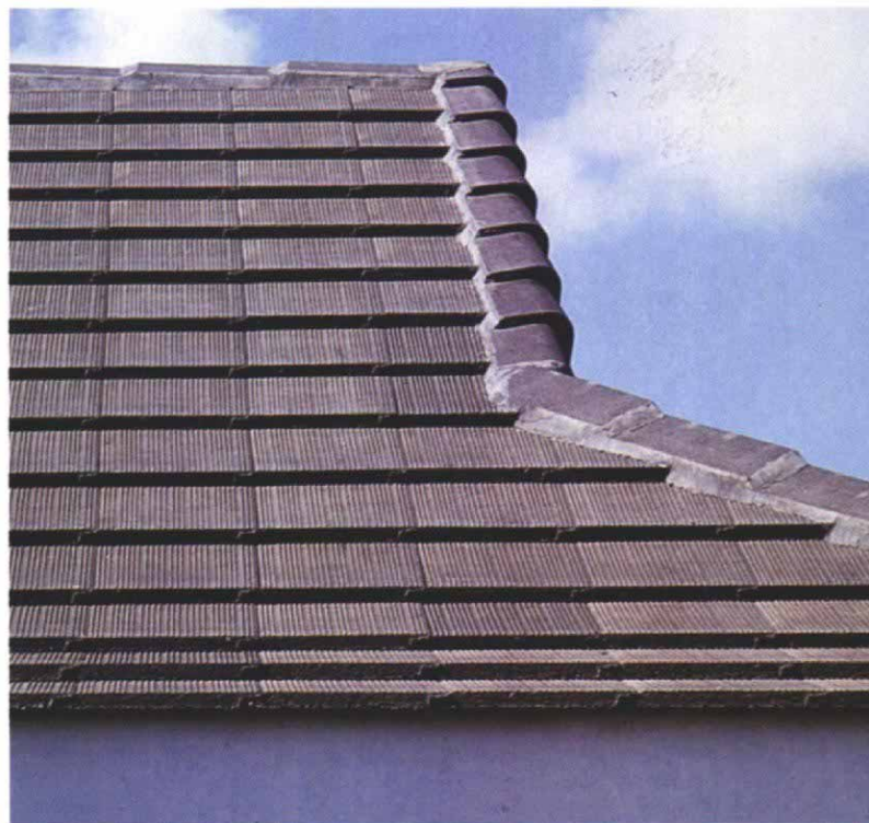
Flat tiles can be colored and textured to resemble traditional roofing materials such as slates, or the wooden shakes suggested by the dark, striated patterns of the concrete tiles on this roof.
