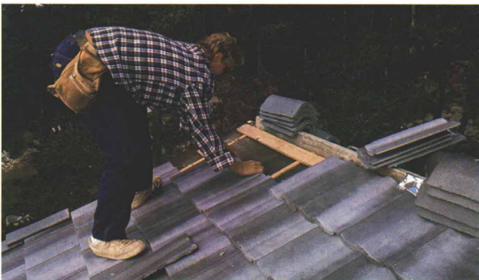
Low-profile concrete tiles. After the roof is felted, horizontal battens are affixed to the roof sheathing. Lugs at the top of the tiles bear against the edge of the battens to hold them in place. In seismic zones and windy areas, the tiles should also be nailed down.
