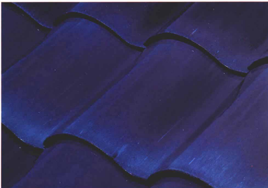
While most tile roofs cap a house in earth-toned silence, the rich colors made possible by using vitreous glazes on ceramic tiles can make the impact of the roof the dominant element in the bearing of a house.
