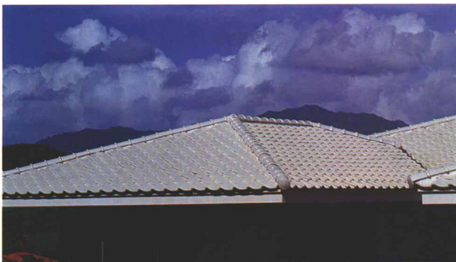
Glazed clay tiles. Tiles made of clay can be finished with baked-on glazes in both custom or stock colors. This Japanese-style roof in glossy white is essentially the same as the interlocking S-type mission tile, but its trim pieces, such as the cylindrical hip starters and the belled ends of its hip and ridge tiles, give it an exotic flair.
