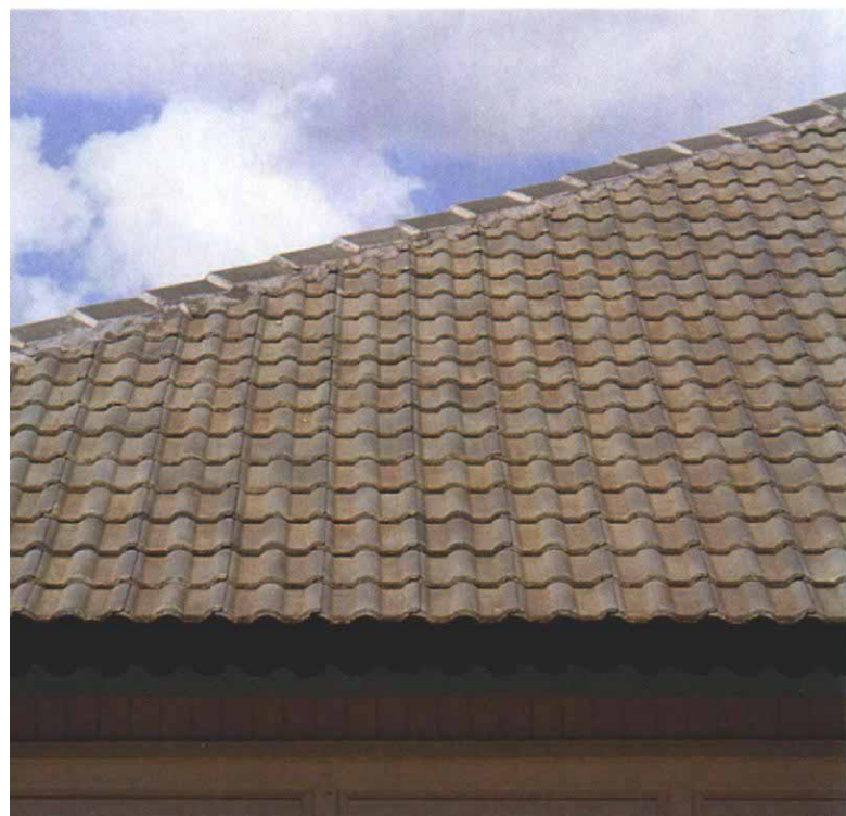
Low-profile tiles are designed to interlock at the edges to keep out the weather. These variegated concrete tiles have been colored with a slurry of cement and iron-oxide pigments.
