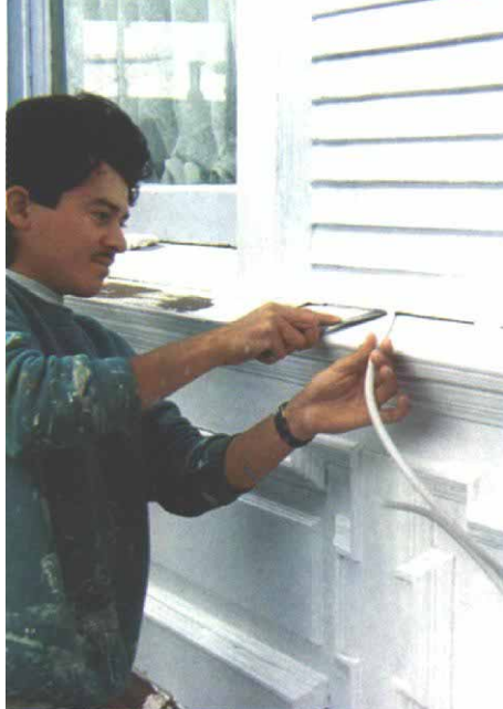
Filling wide cracks. Backer rod is a compressible foam rope that can be squeezed into a crack too wide to caulk. Once in place, the remainder of the crack is filled with caulk.
