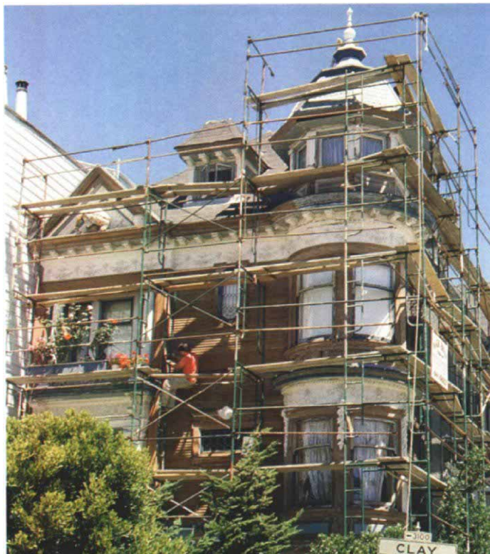
Almost a century old, this Queen Anne Victorian house is decorated with redwood trim and plaster garlands. A job of this scope begins with a thorough cleaning done from a scaffold that allows access to every exposed portion of the building.
