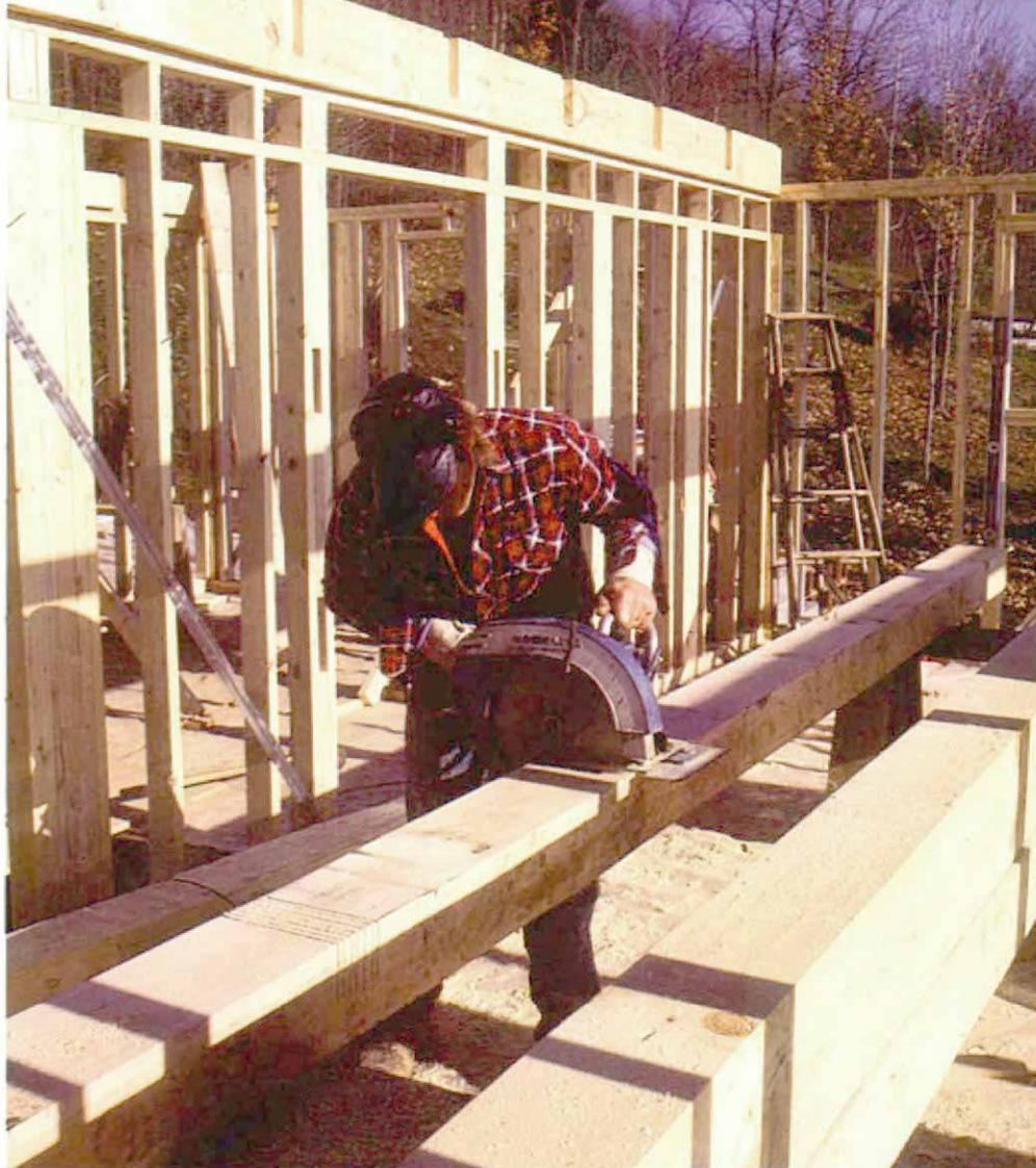
**Notching the rim joist.** Because the joists will actually bear on the stud wall, they don't have to be mortise-and-tenoned into the rim joist, but can engage simple notches cut across the face of the timber. Here the notches are being cut with a 12-in. gas-powered circular saw that the author bought at a yard sale.
