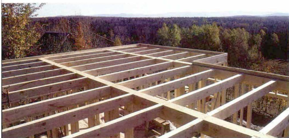
**Joists in place.** Four-by-eight joists are set in their notches and secured with 12-in. spikes driven through the outside of the rim beams and with 20d nails toenailed down into the summer beams. The framing will also be tied together by a floor system above.
