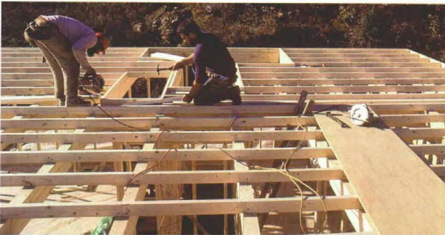
**Making room for pipes and wires.** When the downstairs ceiling is the upstairs floor, it complicates the routing of wires, pipes and ducts. Nash solves the problem by installing 2x4s on edge across the tops of the timbered ceiling, leaving room for mechanicals, then covers the 2x4s with plywood.
