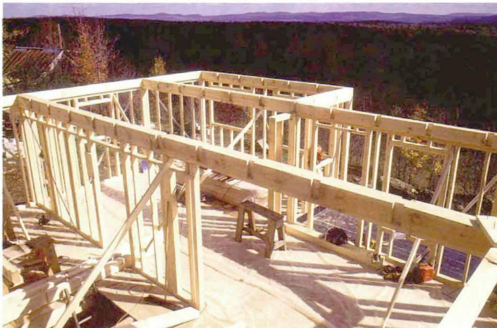
**Rim and summer beams.** In place of the rim joists of conventional platform framing, 6x8 rim beams are set on the exterior walls, with 8x10 summer beams supporting the joists at midspan.
