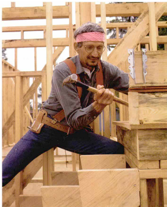
Traditional winder construction methods apply treads and risers to short stringers. Production methods offer a quicker approach.
