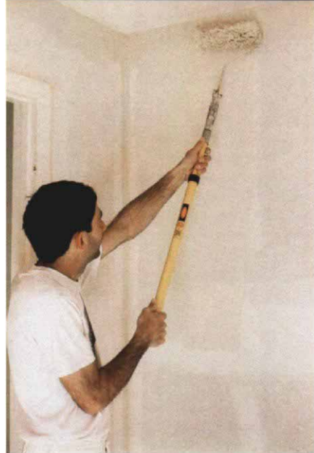
Beginning at the left corner on a wall, the author levels out a patch of flat latex paint. The cut-in is wide enough to allow him to stop the roller within a couple of inches of the ceiling.
