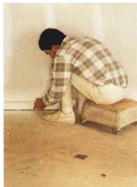
Scooting along on a roller stool, Papa can quickly tape baseboards without putting a strain on his back or his knees.
