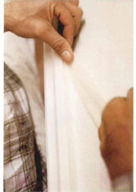
Once the wall paint has hardened for a couple of days, the tape can be peeled away from the trim. Angling the tape toward the wall can help cut down on the amount of tearing.
