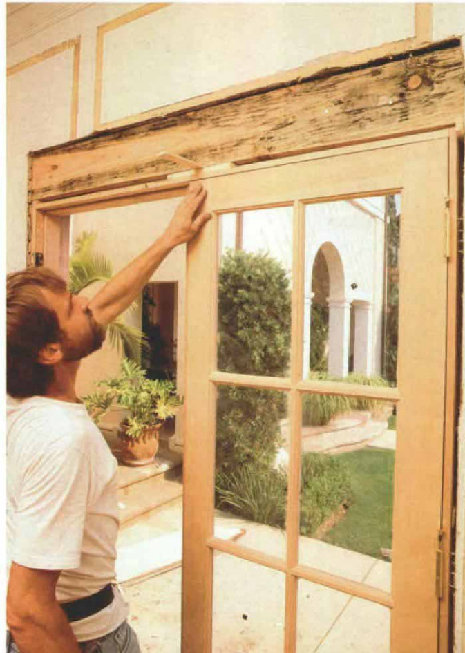
The jamb and doors are brought into square with one another by inserting shims and blocks between the trimmers, header and the jamb.
