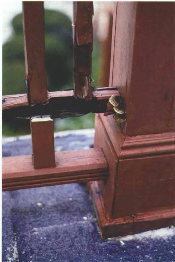
Mushrooming problems. When fungi sprout from railings, it's a rotten sign. Pictured here is a close-up of the railing the author was hired to replace.
