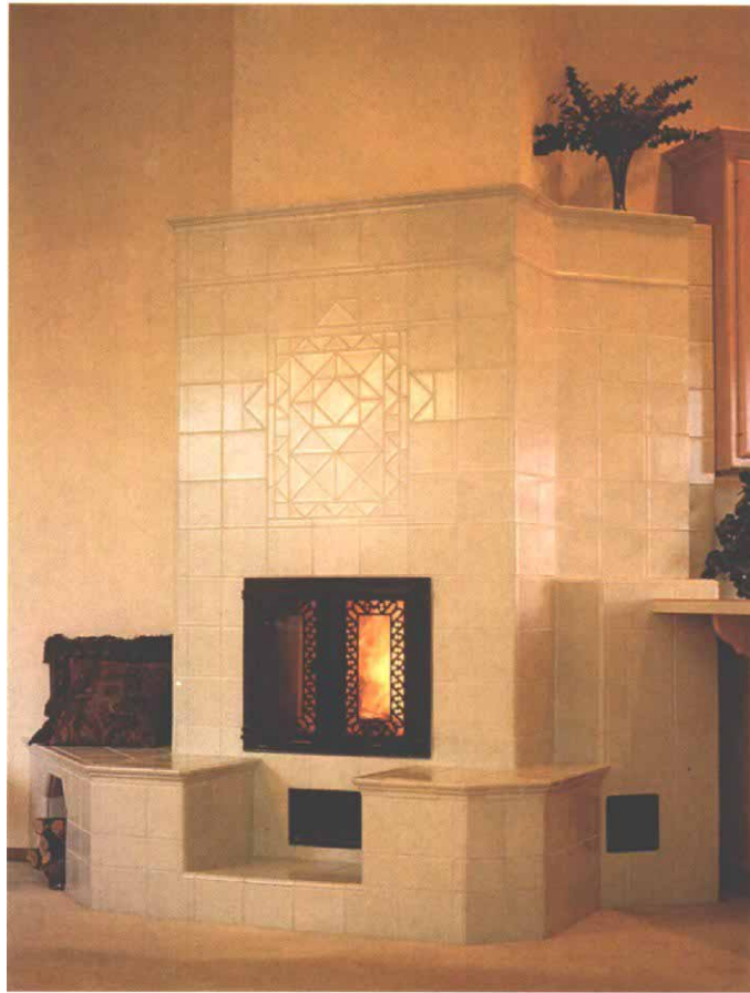
Patterned after the typical Finnish masonry heater, this energy-efficient, clean-burning fireplace can be the focal point of a home.
