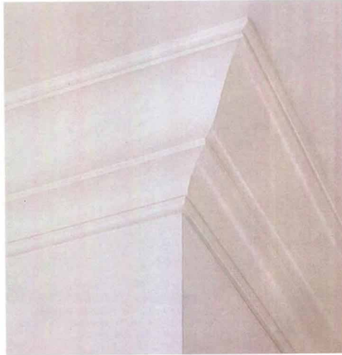
Joined at the shadowline. Wide crowns, which appear to be made of a single molding, can be made by running related profiles adjacent to one another. Any gaps between the two are caulked prior to painting.
